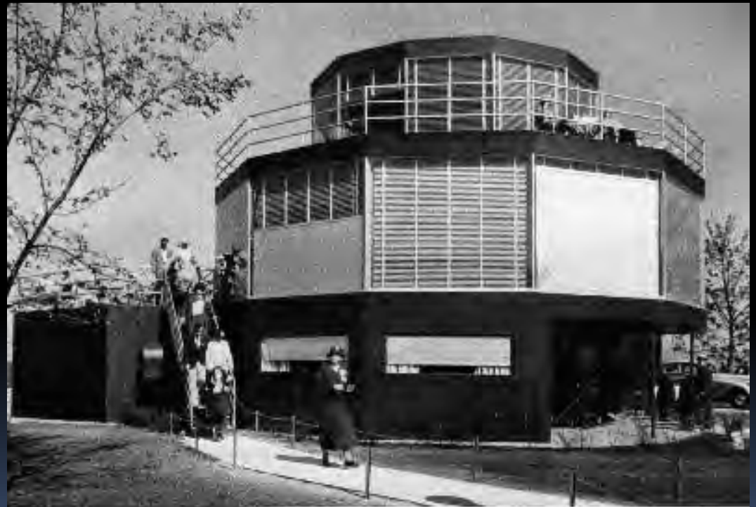
THE HOUSE OF TOMORROW (STEEL AND GLASS)
